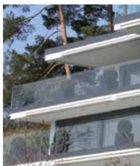
Balustrade de balcon
