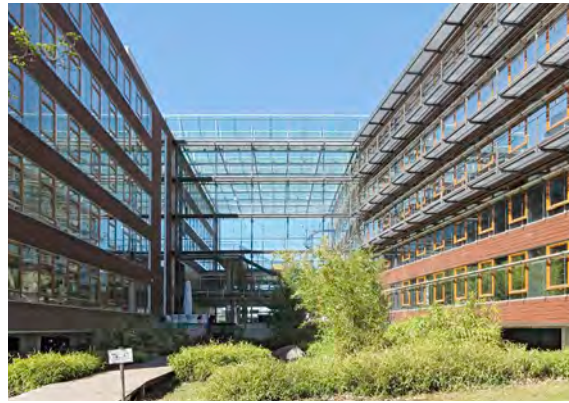
In green inner courtyards or areas of buildings which are enclosed from multiple sides, the risk of collision with glass surfaces increases. Vegetation attracts birds flying over the sea of buildings, but once they are inside they can have trouble taking off at a steep angle and flying away.
