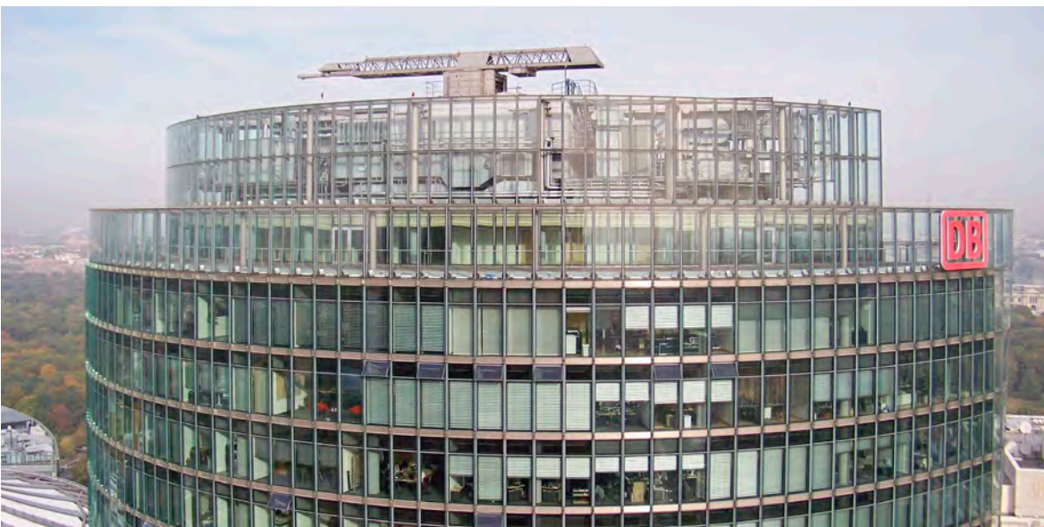
Glass parapet several metres high at the top of a skyscraper. Birds not only collide with the glass from the outside, but also hit the panes from the inside after ending up within the enclosed area.
