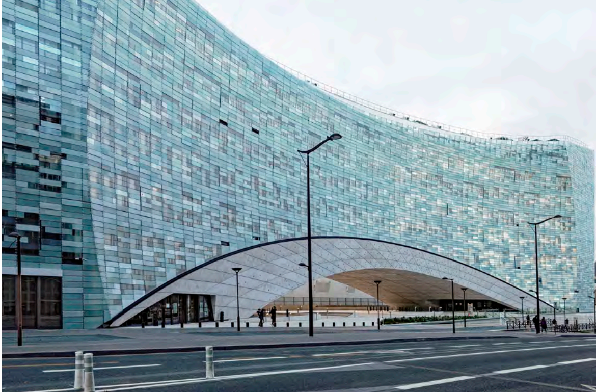
The façade of the headquarters of Le Monde in Paris, designed by Snøhetta, is made up of more than 20,000 glass elements. These vary in structure and transparency and are arranged in such a way that they maximise the light in the offices and provide views to the outside in the right positions.
