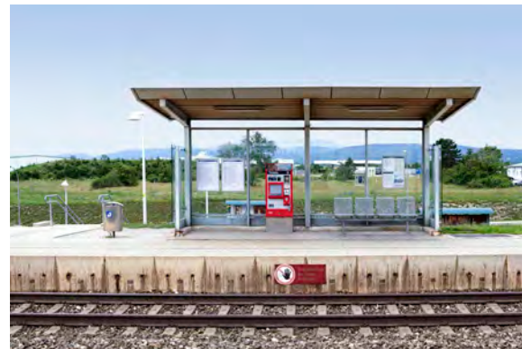
Public transport shelters are often made of glass without considering safety measures for birds.
