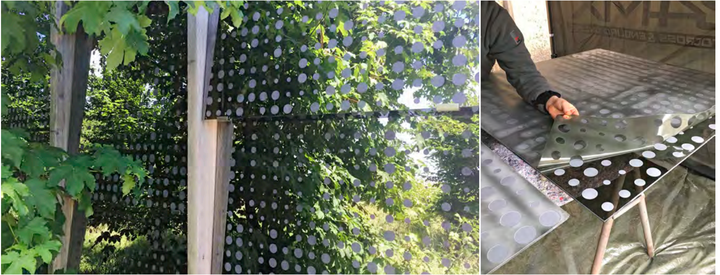
This façade in Scharnstein, Austria was improved by sandblasting. To prevent bird collisions, the individual highly reflective glass panes were removed and then modified on site by a process of partial sandblasting ('punch card' dot grid in varying diameters).
