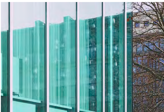
These collision marks clearly show that tinted glass offers no protection against collisions.
