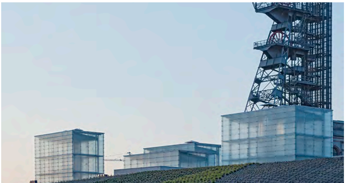
At the Silesian Museum in Katowice, cubes with a façade of etched glass provide the underground museum rooms with daylight. The abstract glass cubes by the architectural firm Riegler Riewe blend harmoniously into the ensemble of existing historical buildings.
