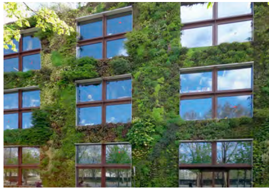
Façade greening on the Musée du Quai Branly in Paris. Such measures, implemented to support biodiversity and improve the city's climate, must go hand in hand with efforts to prevent bird collisions.
