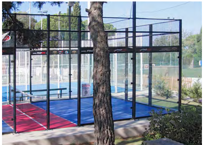
Padel tennis courts are sometimes surrounded by transparent plexiglass. Evidence from Spain, Italy and other European countries has shown numerous bird collisions with these walls.
