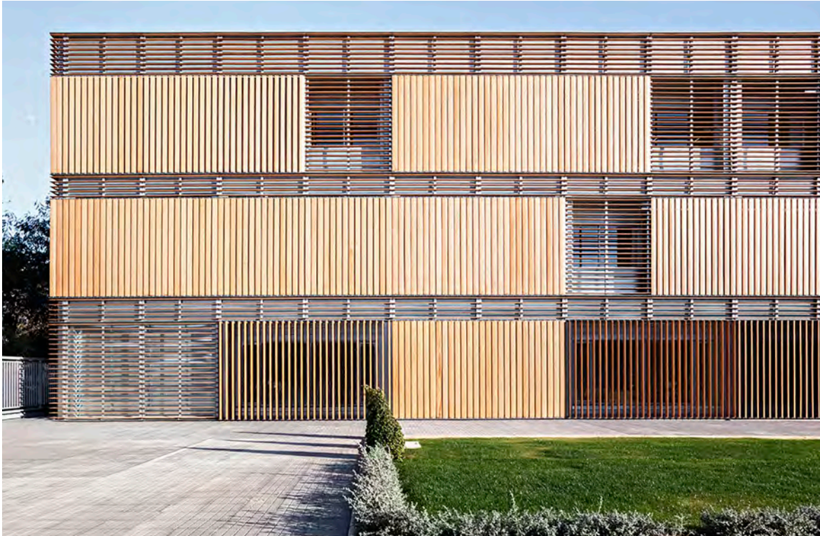
In the west block of the Centre d'Idiomes de la Universitat de València, Spain, by Arkitera SLP, the combination of fixed and movable sunshade slats defines the structure of the façade.
