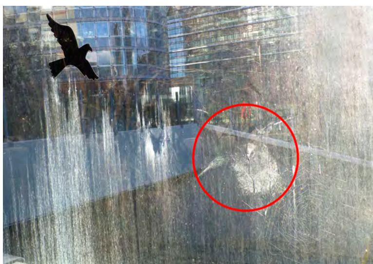
Collision marks are repeatedly found directly adjacent to silhouettes of birds of prey. Cleaning windows less frequently also provides no protection against bird collisions.
