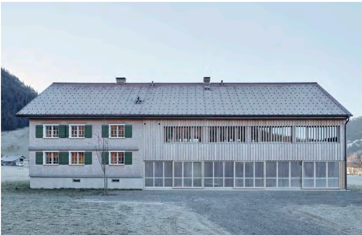
When renovating and repurposing the heritage building 'Großenbündt' in Hittisau, Austria, the architects Gruber Locher Architekten provided light to the ground floor by using semi-transparent materials. While the traditional grid windows of the residential wing were retained, the structure of the traditional wooden façade was echoed in the wooden slats over the long ribbon windows on the upper floor. Birds can easily recognise these materials and structures.
