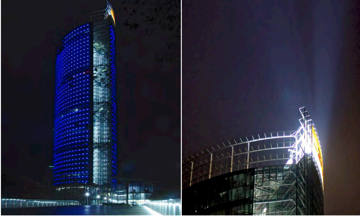
Effect lighting behind the outer glass façade and illuminated company logos on the roof lure migratory birds to their death at the Post Tower in Bonn. Exposed advertising panels, construction cranes, aviation safety lights, and other light sources high above the ground lie in the flight path of migratory birds and present an often-underestimated threat.
