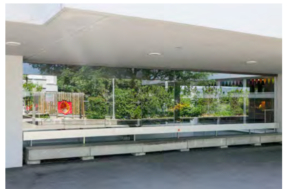
Although the building protrudes by several metres, clear reflections are still visible on the windows. Shadows cast on windows do not eliminate reflections.
