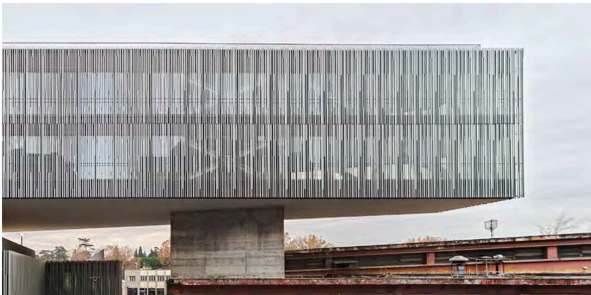
The Città del Sole ('Sun City') in Rome, by Labics, is a multipurpose facility with public and private functions. Both the design of the façade's aluminium panels and the translucent glass slats on the various buildings provide protection from the sun and for birds in equal measure.
