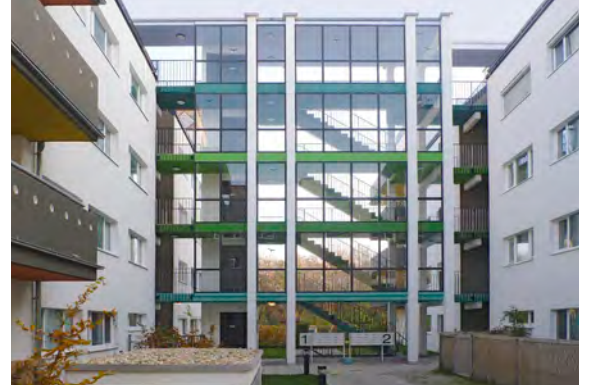
The danger posed by glass walls and passageways is exacerbated when buildings on either side force the birds towards the obstruction.
