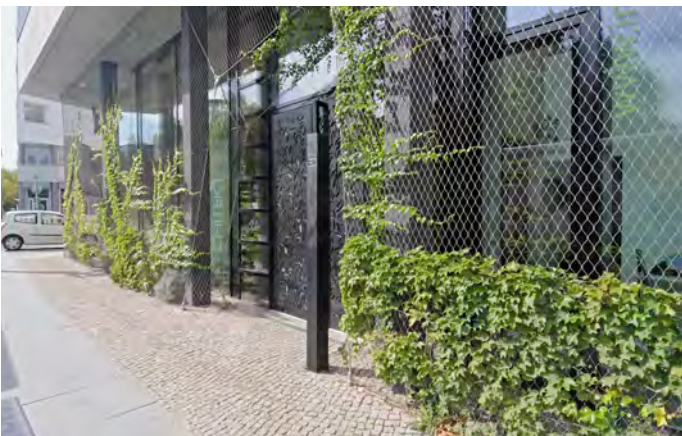
Steel mesh, often used to grow plants on buildings, can also be used for bird protection if the cables are thick enough. For the Engeldamm Passive House (PHED) in Berlin, designed by scarchitekten joerg springer/robert mieth, this form of façade was planned from the outset. Depending on the nature of the façade, however, this type of netting can also be retrofitted.
