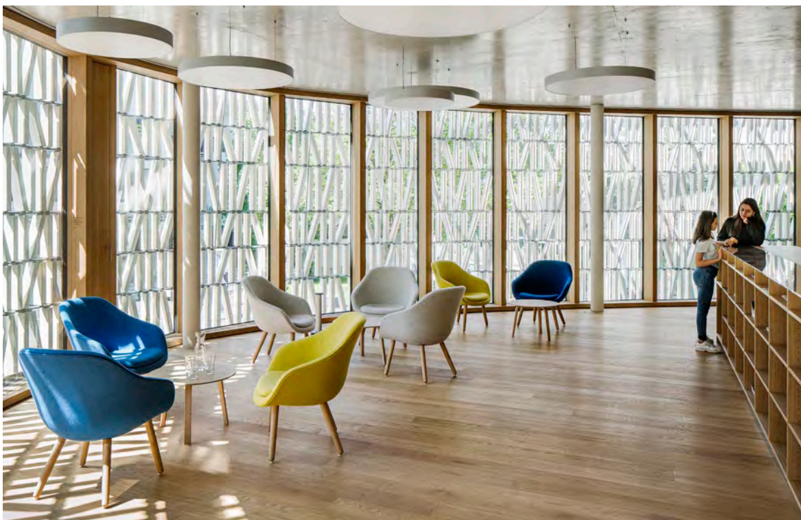
The oval-shaped glass pavilion of the Dornbirn Municipal Library, Austria, by Dietrich | Untertrifaller, is wrapped in a structure of 8,000 prefabricated ceramic elements. Arranged vertically and diagonally, the sunshade ornaments are reminiscent of bookshelves and provide pleasant natural light inside.
