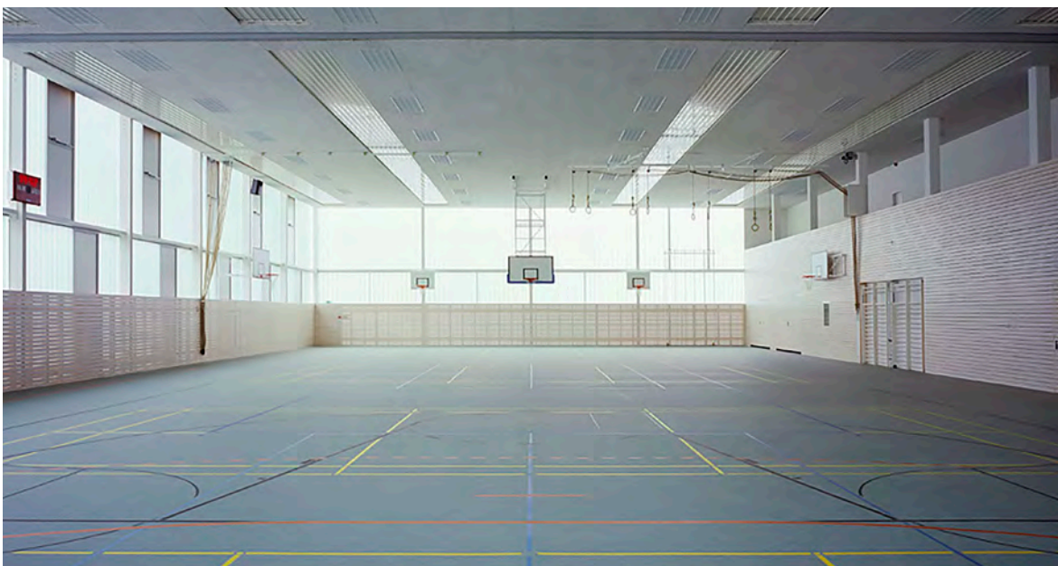
The building envelope of this ball sports complex in Ingolstadt, Germany, by Fink+Jocher, consists of a channel glass construction filled with translucent thermal insulation between its two glass profile shells. This enables sufficient light to enter without causing disruptive shadows on the court.
