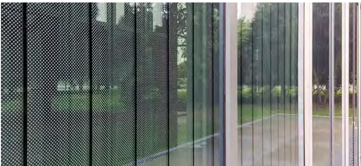
Bauhaus Museum Dessau: Despite a coverage rate of 30%, the fine dot grid is unsuitable for bird protection due to its low recognisability for birds. The façade was therefore retrofitted with black stripes.
