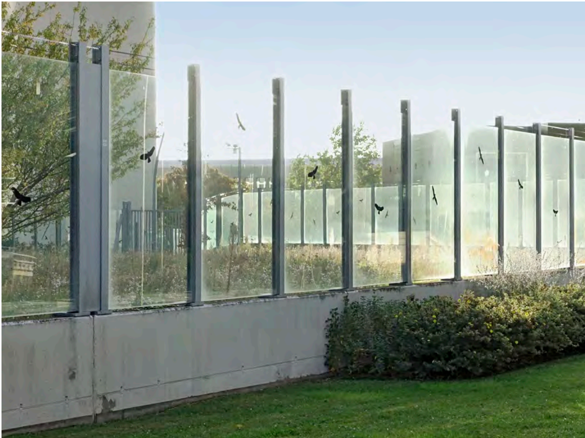
Stickers of the silhouettes of birds of prey usually indicate that collision is a known issue in this location. However, they are not effective and should not be used, as collisions will continue to occur in direct proximity to the stickers. Instead, tested markings that mark the entire glass surface should be used.
