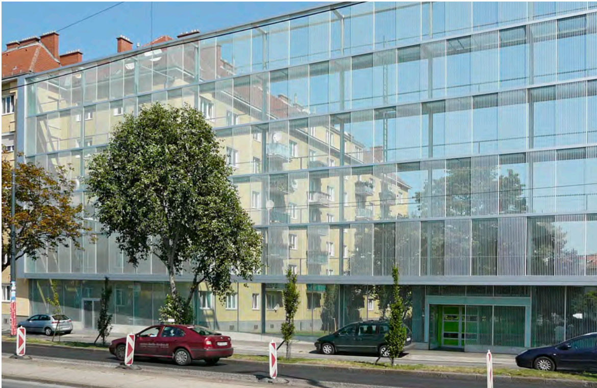
The bird protection pattern used in this noise barrier by Treusch architecture in Theodor-Körner-Hof in Vienna deliberately emphasises its three-dimensional structure.
